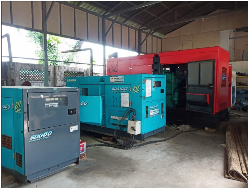
Figure 3-14 Diesel Generators
