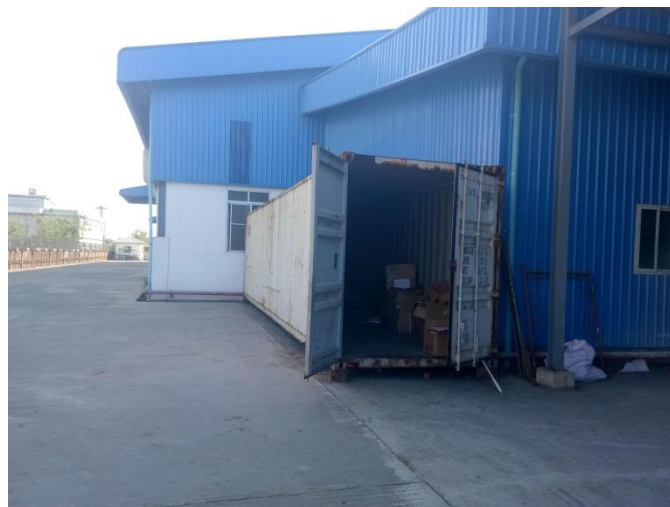
Recycle Waste Dumping Area
