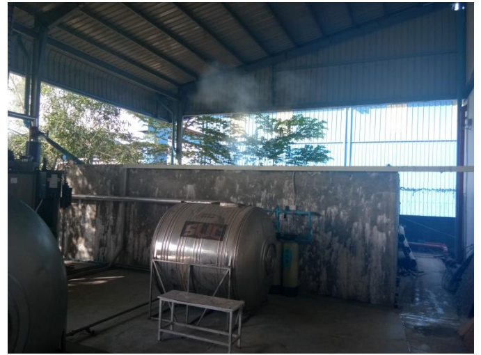
Fire Water Tank
