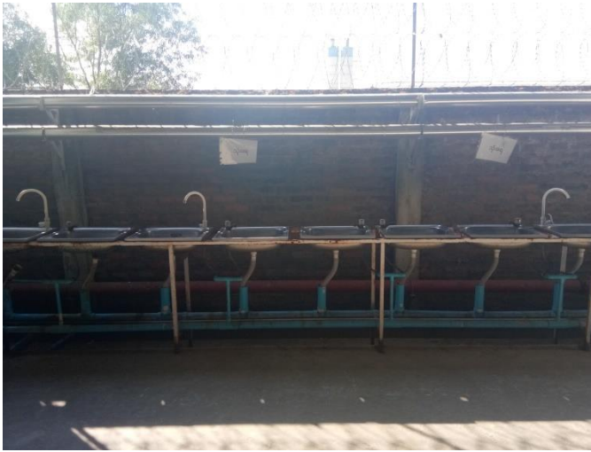
Sink for Employees
