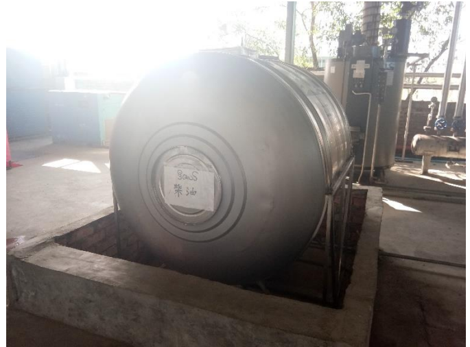
Diesel Fuel Tank
