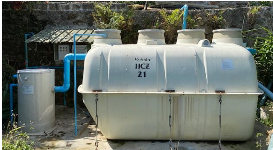
Figure 5.10. Installed Kubota Waste Water Treatment Plant at project site
