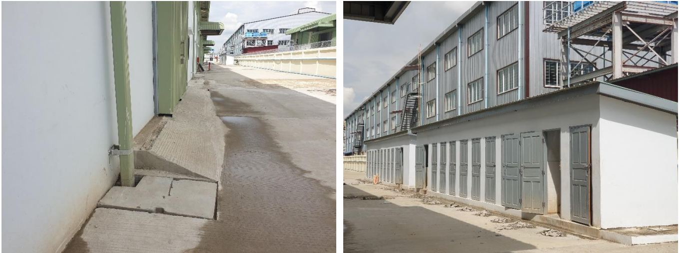
Figure 3-12 Drainage and Toilet facility
