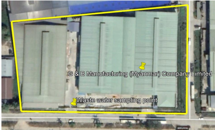
Figure 20. Waste Water Sampling Point
