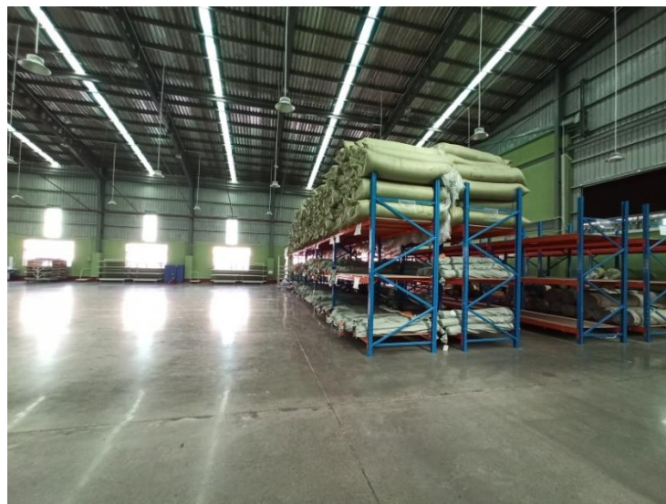
Figure 9. Raw Material Storage Area
