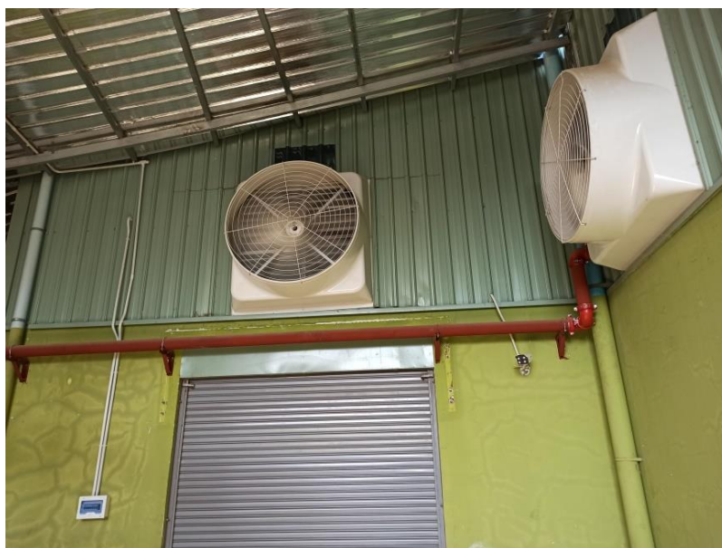
Figure 26. Exhaust Fan are Installed for Ventilation
