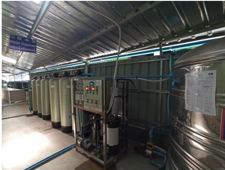
Figure 18. Drinking Water Treatment System is Installed for Drinking Water
