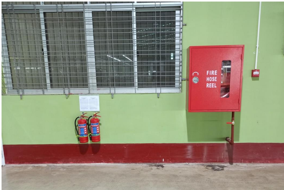
Figure 39. Fire Extinguishers, Fire Hose Cabinets and Fire Alarm Is Provided For Emergency Cases
