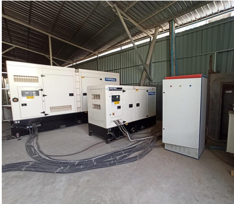
Figure 13. Generator Storing Area
