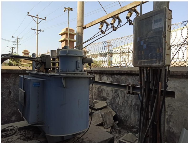
Figure 12. Automatic voltage stabilizer Storing Area
