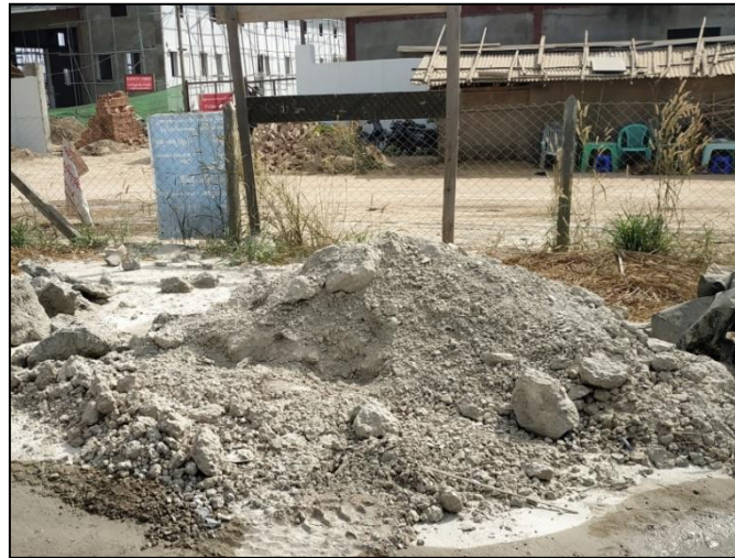
Figure 5.15 Concrete Waste Area to be Recycled for Landfill
