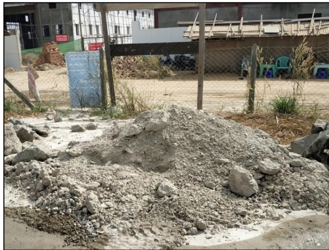
Figure 7.3 Concrete Waste Area to be Recycled for Landfill
