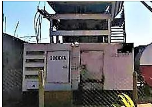
Figure 5.12 Photos of Generators
