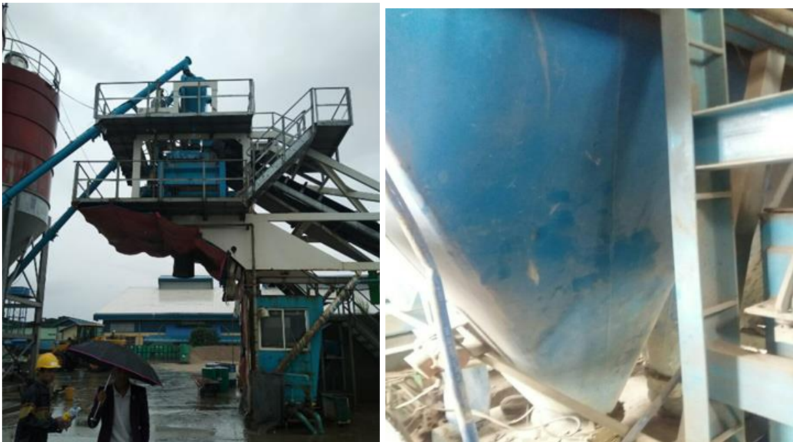
Mixer and Cement Box
