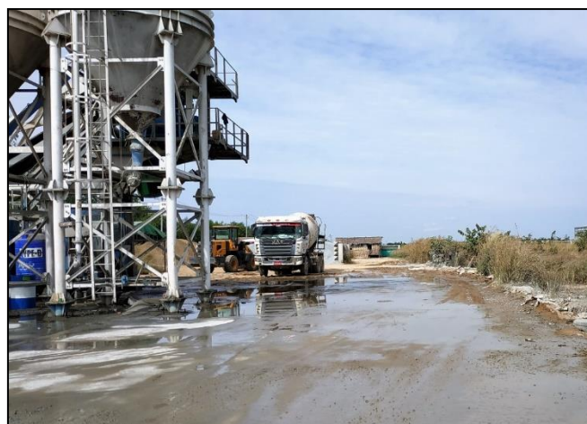
Figure 5.9 Photos of the Batching Plant
