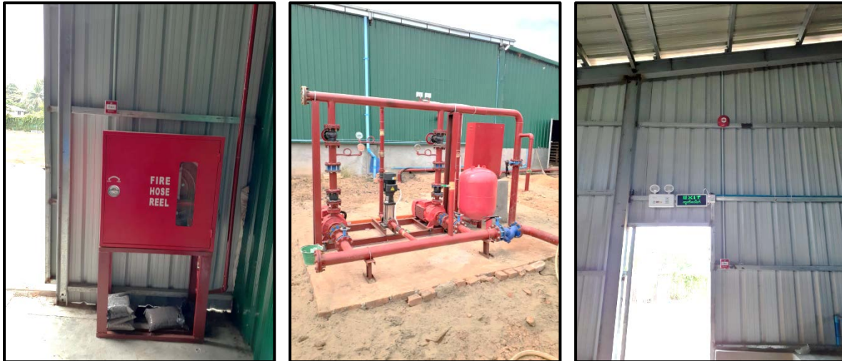
Figure 9-2 Firefighting Equipment Used in Factory
