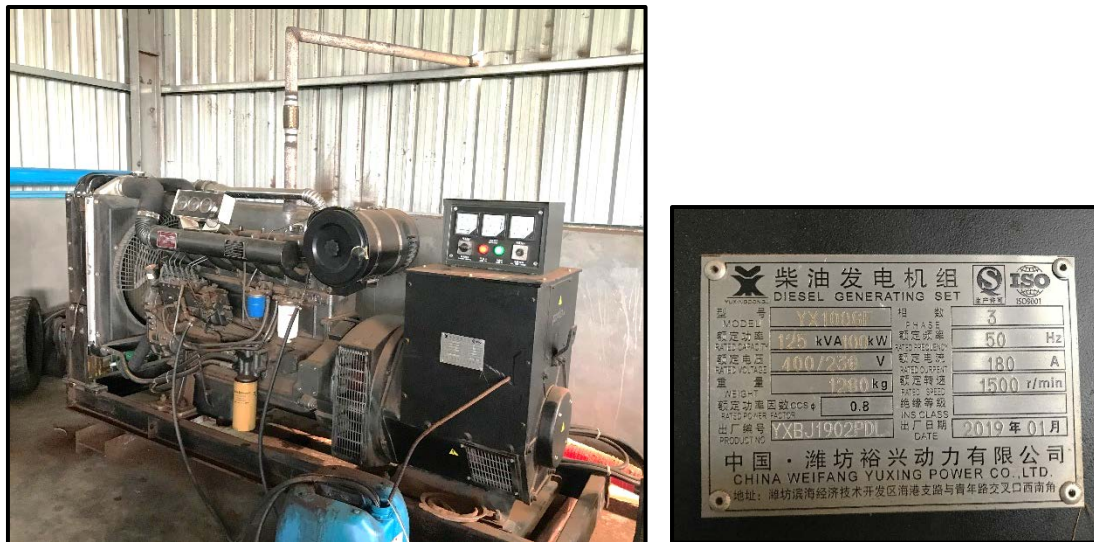
Figure 2-21 Generator for Emergency
