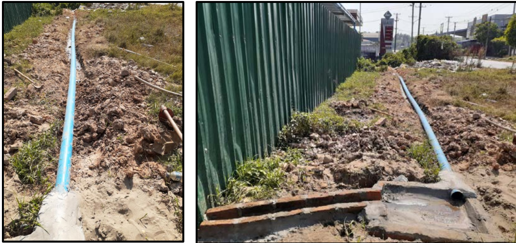
Figure 2-25 Drain around the Factory
