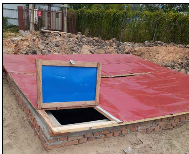
Figure 2-23 Underground Water Storage Tank
