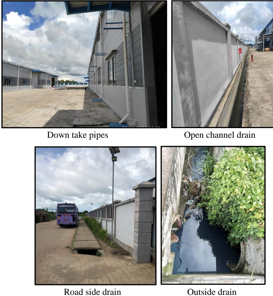
Figure 4-37 Storm Water and Drainage System
