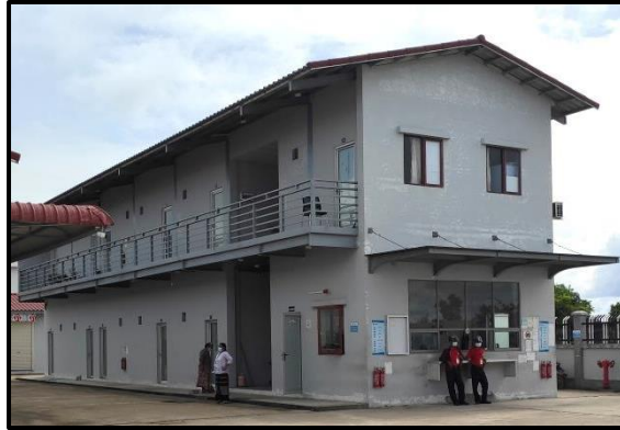
Security House and Hostel
