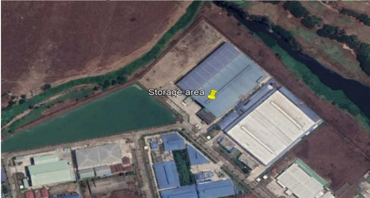
Figure 5.6: Ambient air monitoring at Storage area
