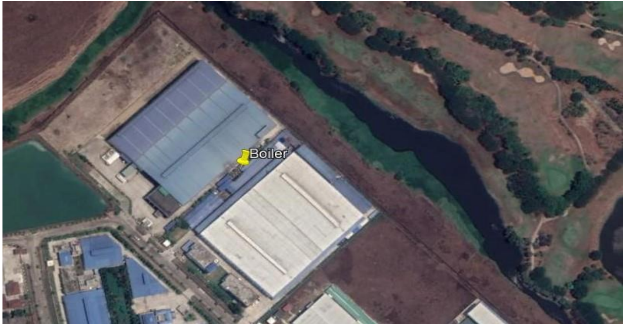
Figure 5.8: Ambient air monitoring near by the boiler
