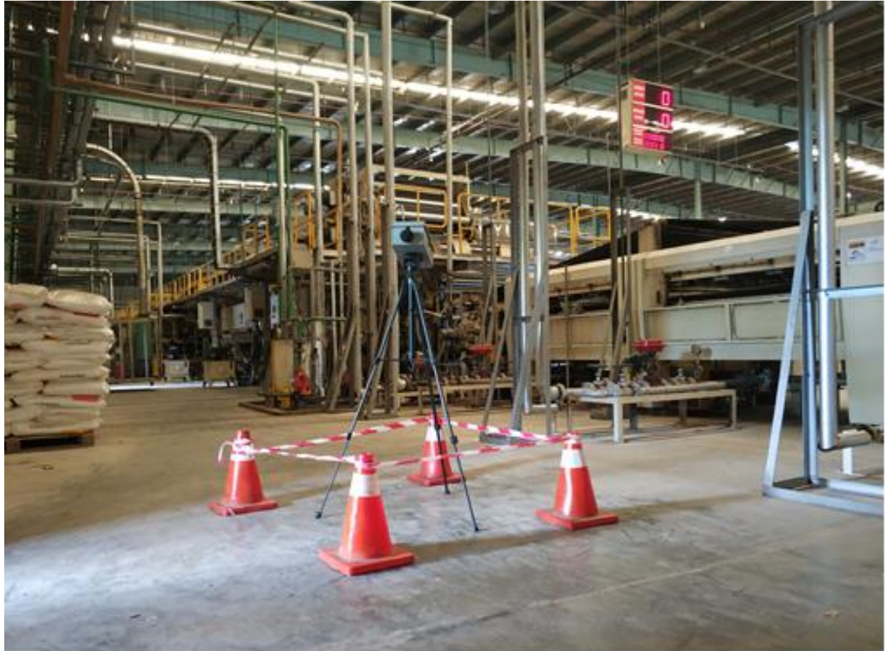
Figure 5.24: Noise monitoring station at factory production area
