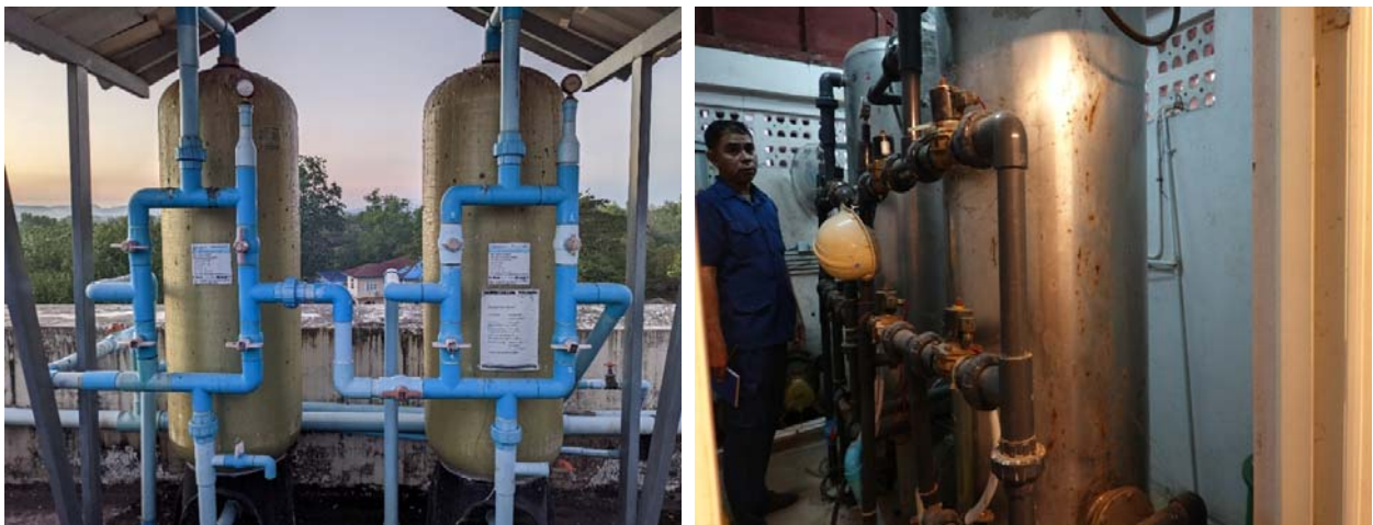
Figure 1-7 Reverse Osmosis System (RO)
