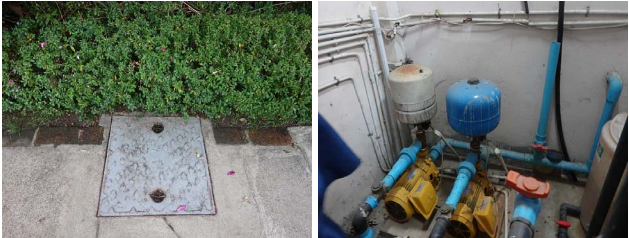
Figure 1-6 Domestic Water & Filtration System
