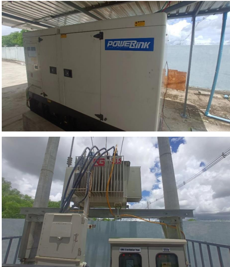
Figure 7. 1000 KVA Transformers And 315 KVA Diesel Generator for Electricity Supply
