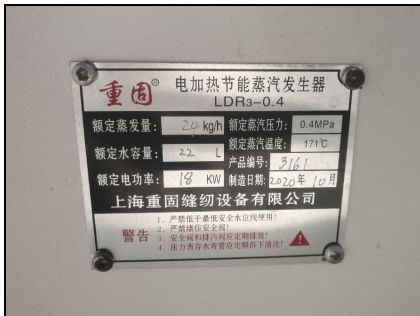
Figure 3-11 Photos of Electric Boiler for Ironing Section
