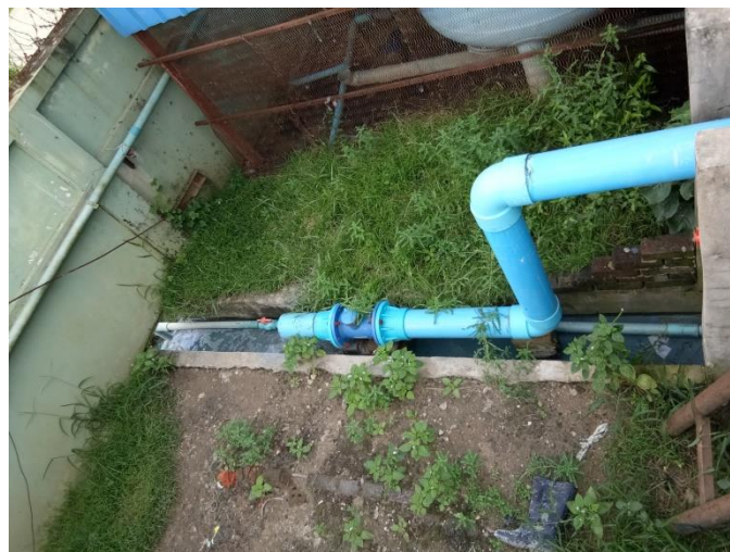
Water Outlet with filter system
