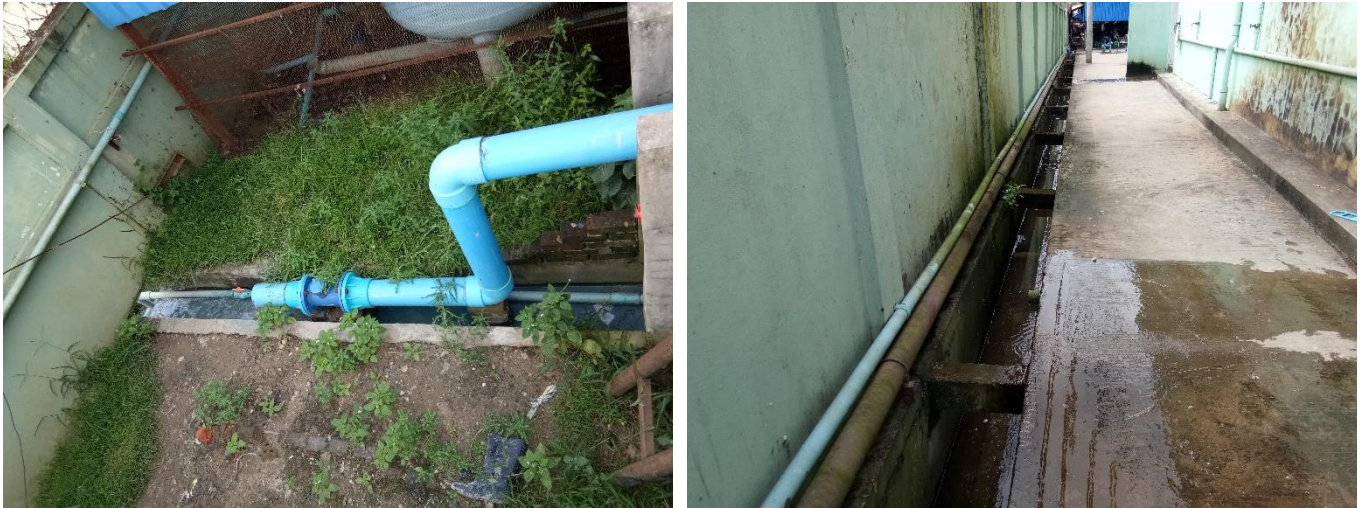
Figure 2-7 Rainwater Drainage in Factory Compound
