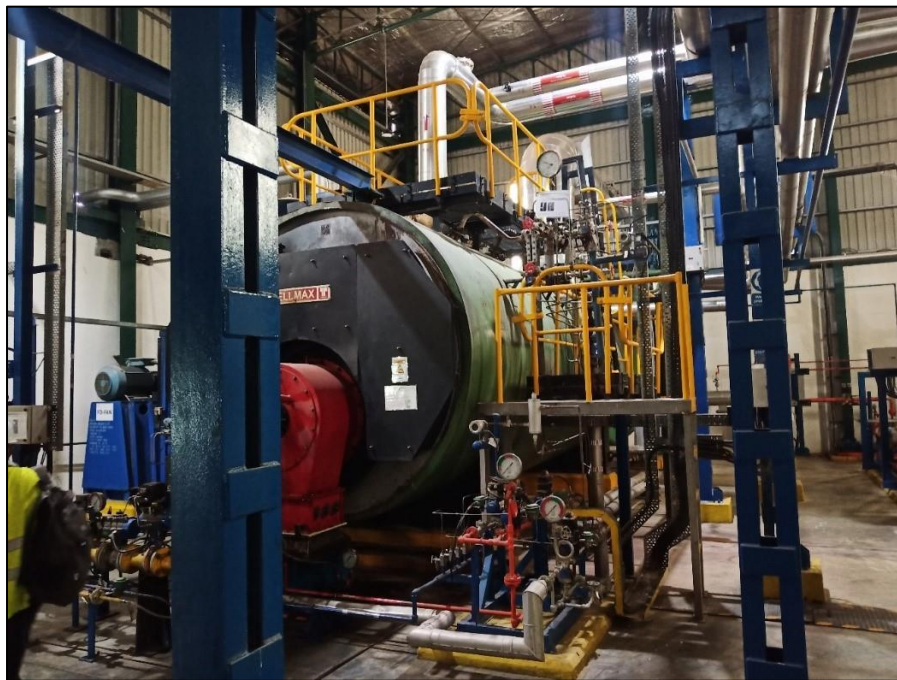
Figure 3-27 Centralized Steam Boiler
