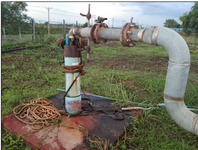
Figure 3-23 Tube Well
