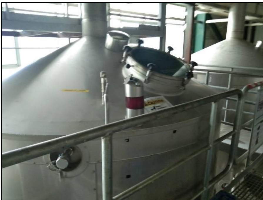
Figure 3-8 Wort Separation Tank
