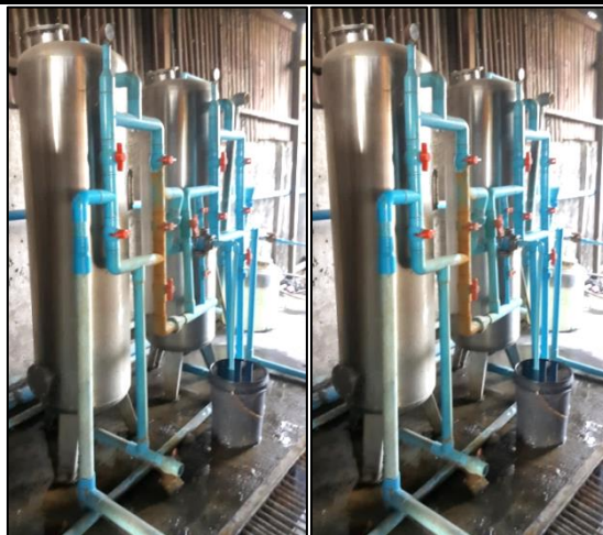
Figure 4-73: Boiler Feed Water Treatment Plant
