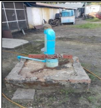
Figure 4-76: The Tube Well and Tube Well Storage Tank
