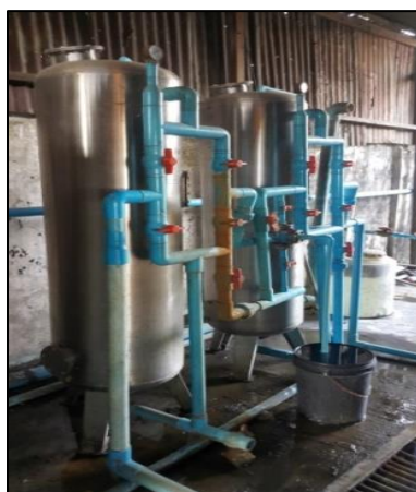
Figure 4-78: The Boiler Feed Water Treatment System
