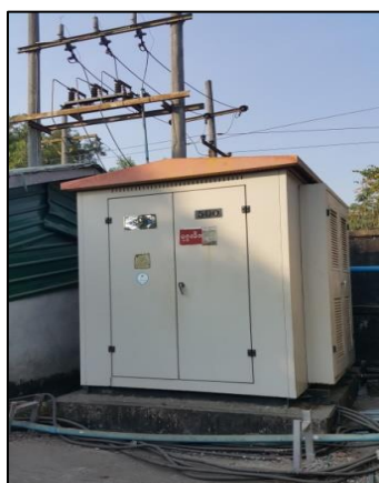
Figure 4-79: Transformer and the Control Panel
