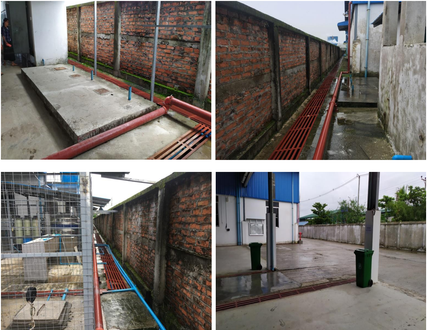
Figure 3-10 Rainwater drainage in factory compound
