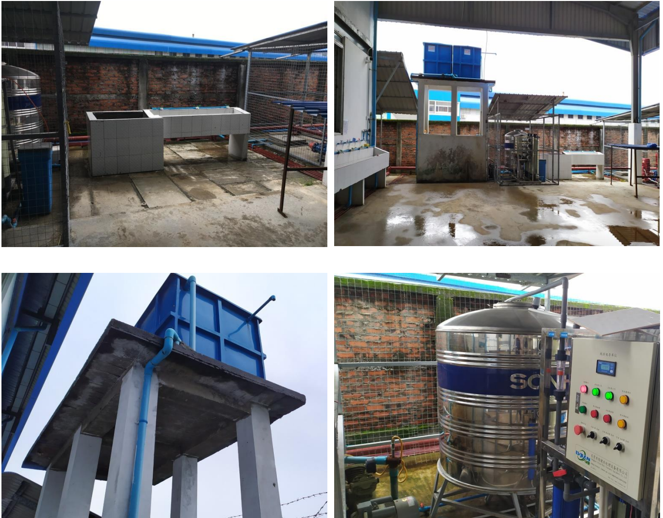
Figure 3-9 Water storage and filtration system
