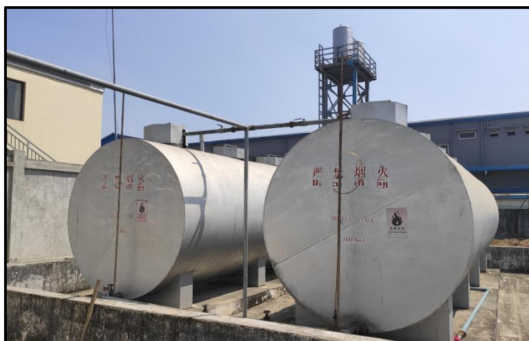
Figure 4-10 Diesel Storage Tanks in Factory-2
