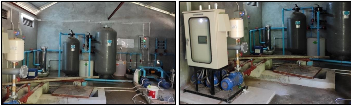
Figure 3-10 Water Treatment System for Domestic Water
