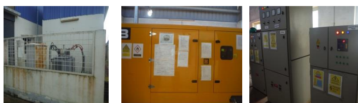
500kVA transformer 400kVA Diesel Generator
