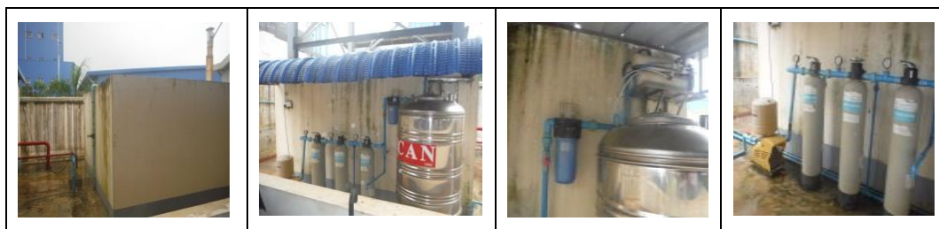
Figure 10 Water Storage tank and RO Water Treatment System
