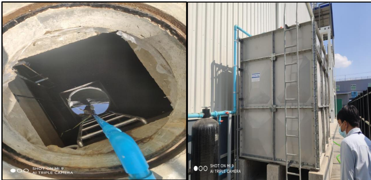
Figure 3.17 A 12000 liter Capacity of Water Treatment Plant Installed
