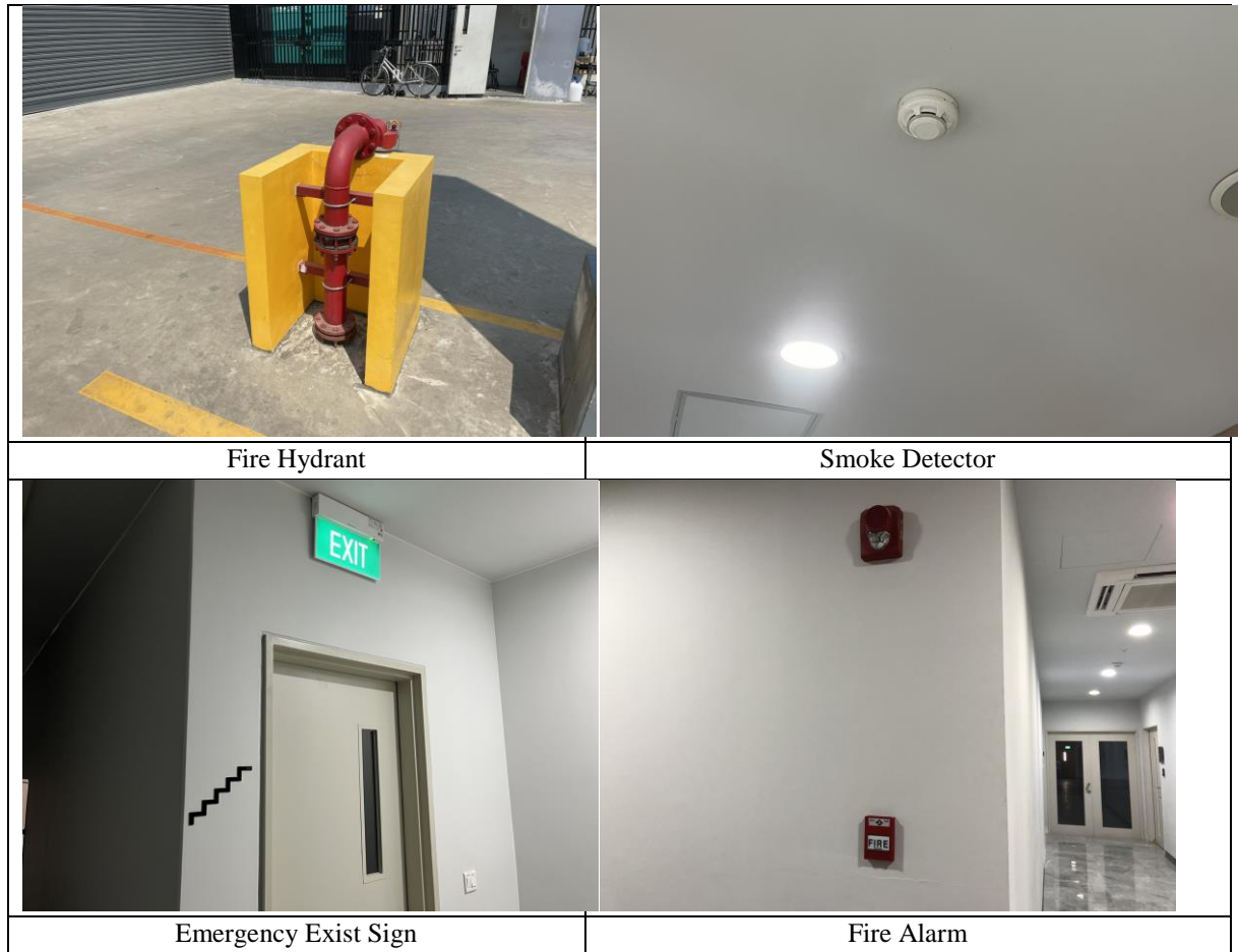
Figure 7.2 Fire Fighting System and Signage
