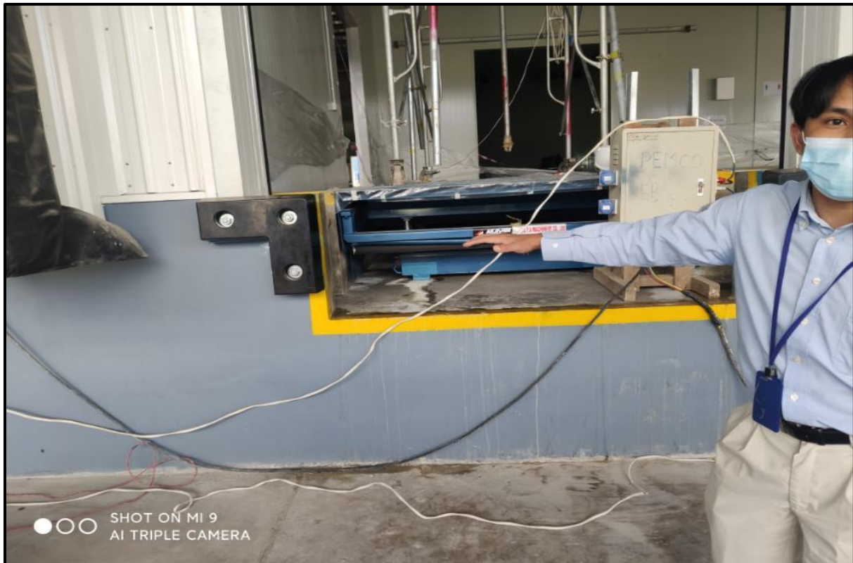
Figure 3.14 Dock Leveler installed in Loading Bay
