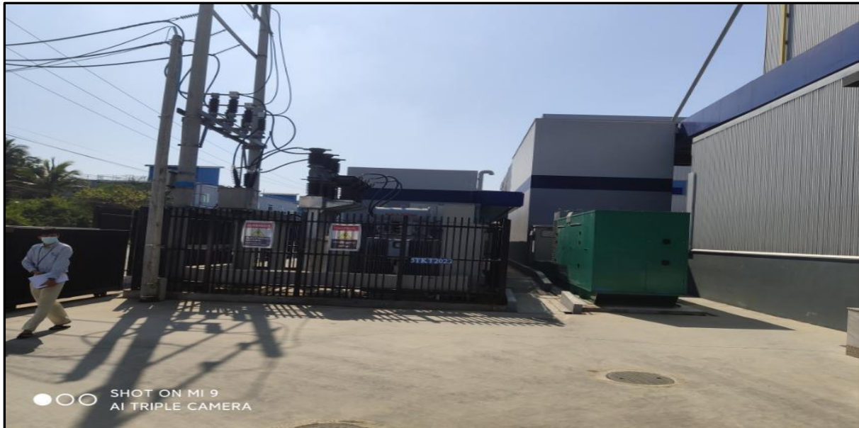
Figure 3.18 A 1000 KVA Transformer Installed
