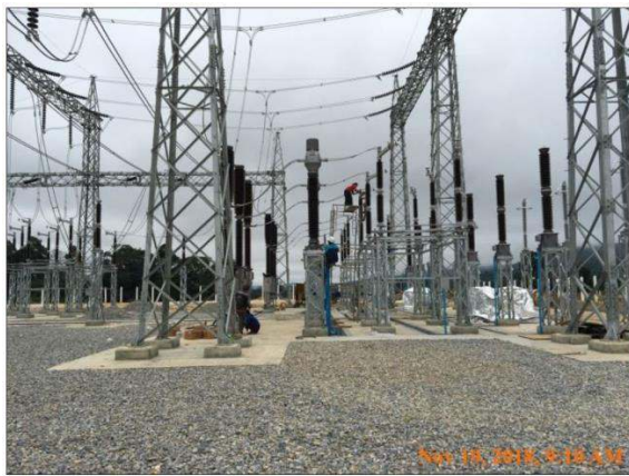
Figure 4-14: Bus Installation Work
