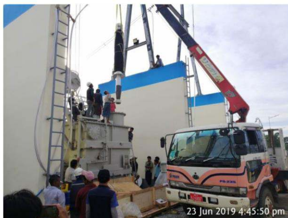
Figure 4-13: Main Transformer Installation Work
