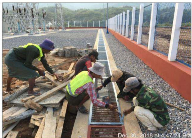
Figure 4-10: Switchyard Drain Work
