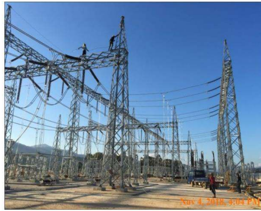
Figure 4-14: Bus Installation Work
