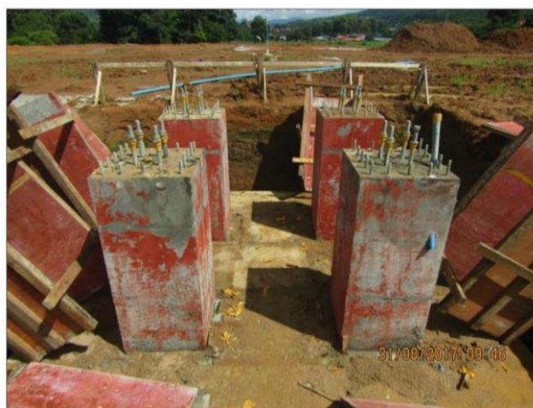
Figure 4-6: Foundation Work (Excavation, Hardcore Filling, Lean Concrete, Rebar Install, and Concrete Work)
