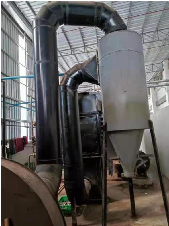
Figure 3-13 Particulate Matter Filtration System of Boiler
