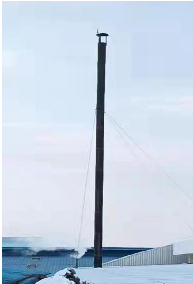
Figure 3-15 Boiler Chimney
