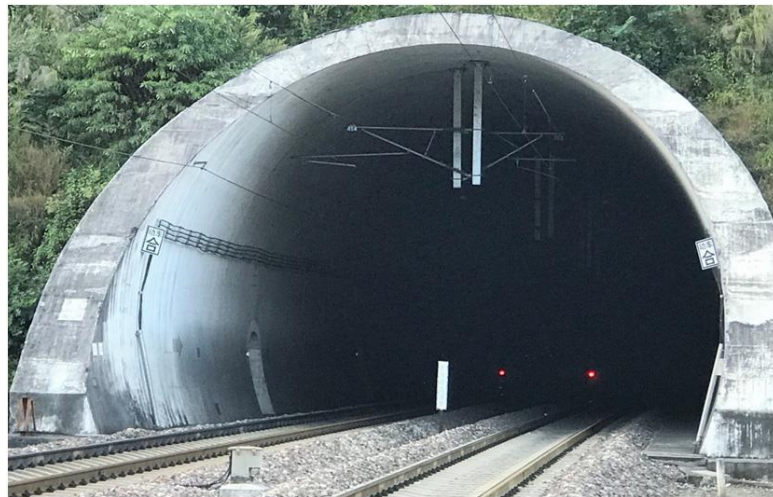
Figure - Drop tube suspension for double-track tunnel
