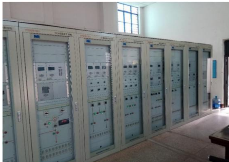
Fig. 4.18 Main control room of traction substation
