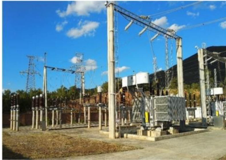
Fig. 4.17 HV incoming side of traction substation
