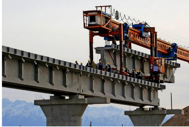
Figure 4.10– Construction of Railway T-beam Erecting by Floating Method
