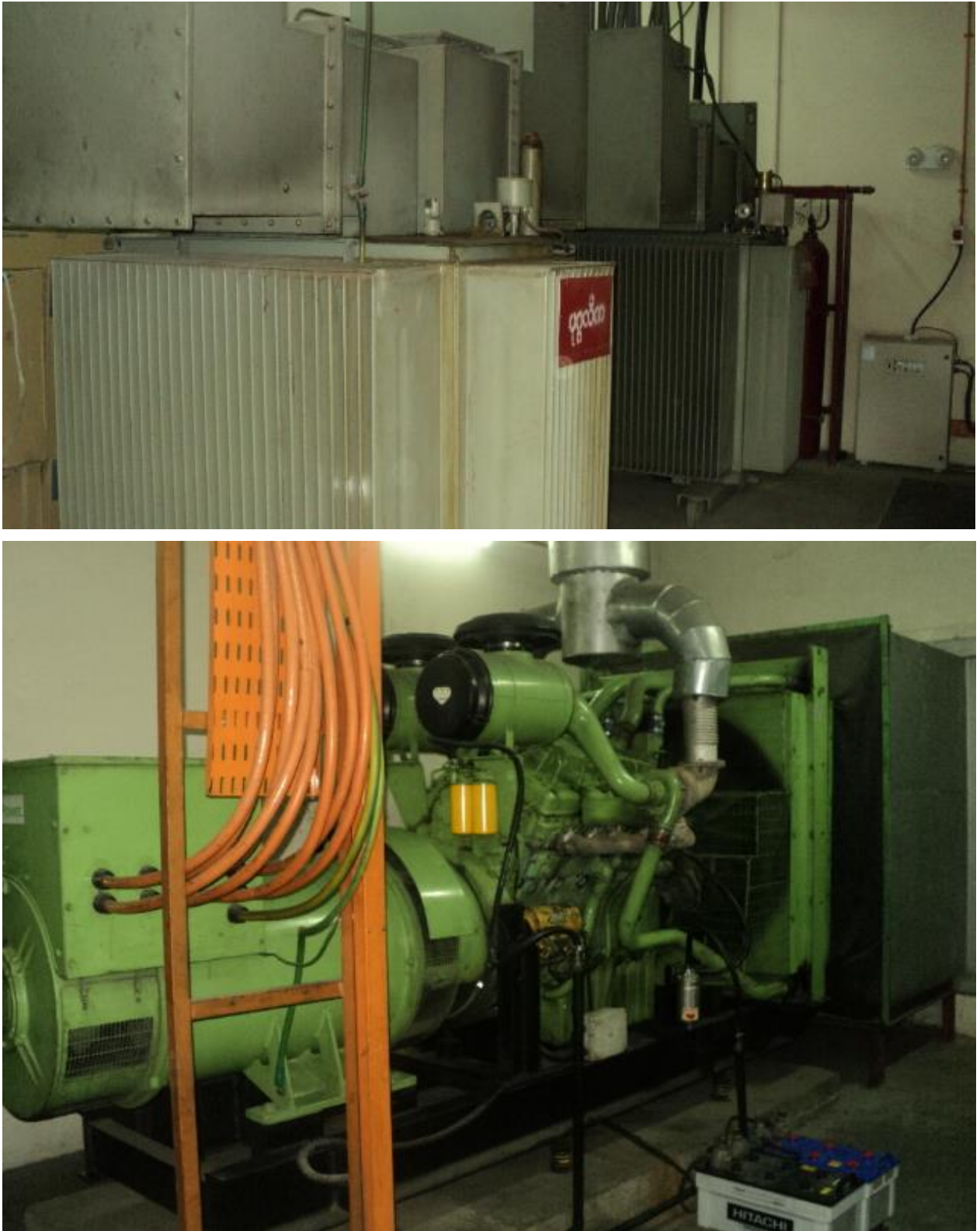
Figure 1.15 Primary and Back-up Power Source of the Mercure Yangon Kaba Aye
