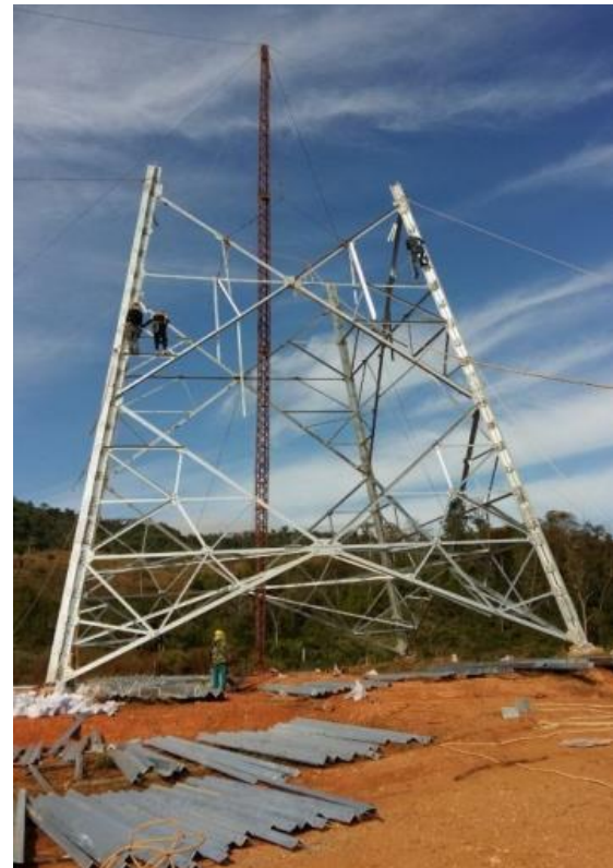
Figure 4.9: Transmission Tower Erection Method (Example Design and Photo)
