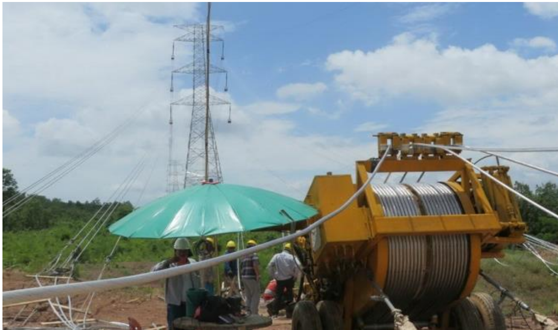
Figure 4.11: Conductor and Ground Wire Stringing Method (Example Photo and Design)
