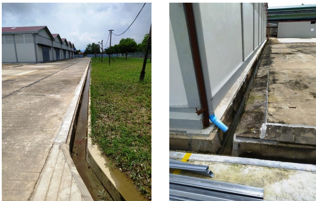
Figure 4.12 Drainage Channels
