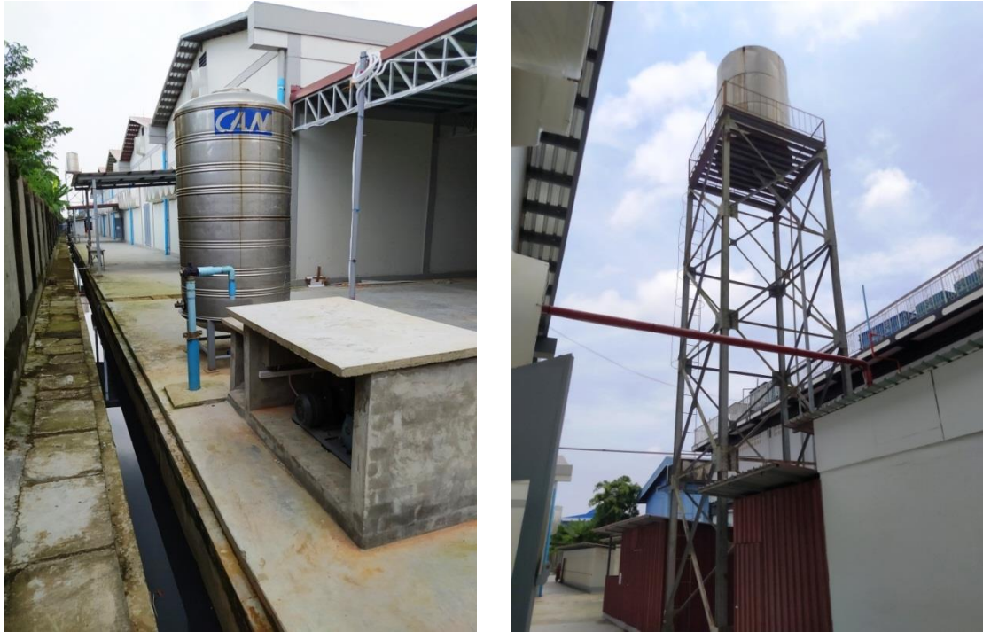
Figure 4.8 Tubes Well and Overhead Tank
