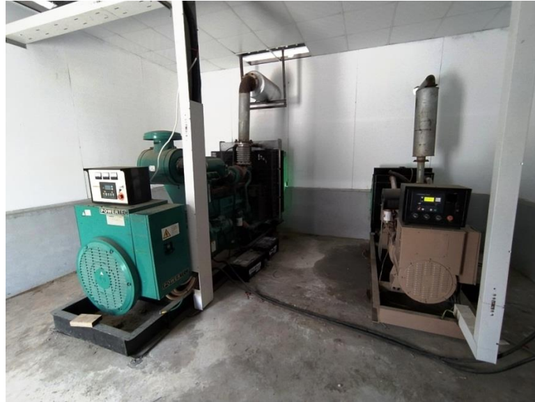
Figure 4.10 Generators
