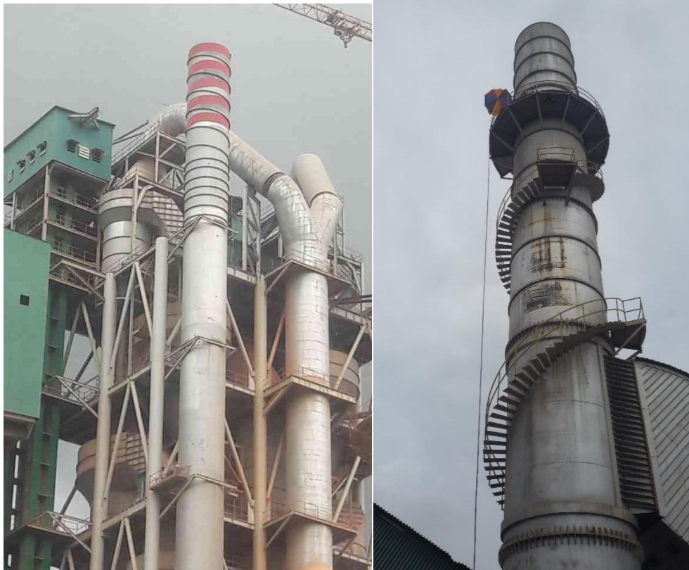
Figure 3.4-23: Preheater Stack (114.5 m) and EP Cooler Stack (40 m)
