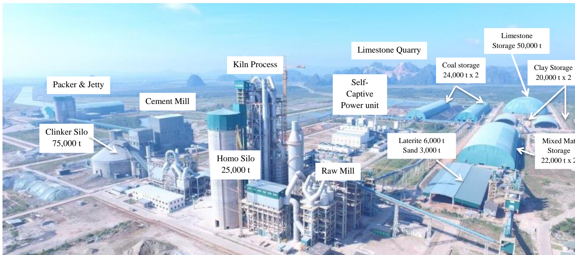
Figure 3.4-25: Plant Layout Overview of Cement Factory Compound
