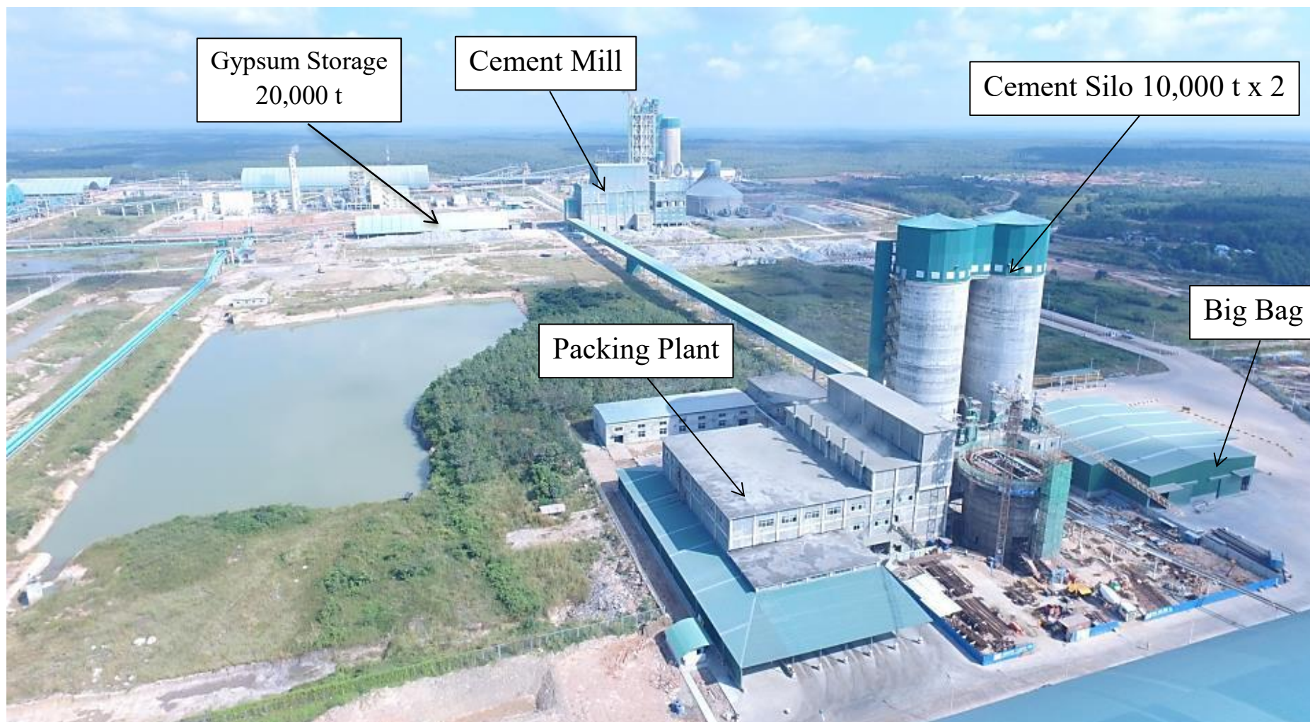
Figure 3.4-26: Plant Layout Overview of Packing Plant and Delivery Area
