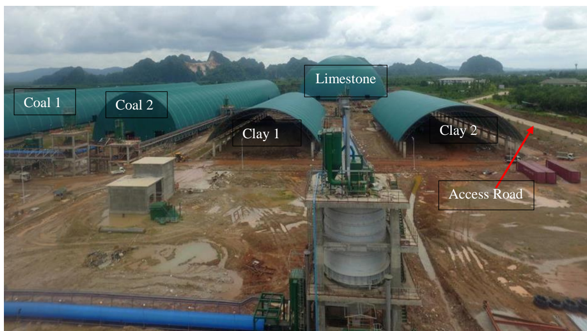
Figure 7.3-7: Raw Materials Storage System Installations in MCL
