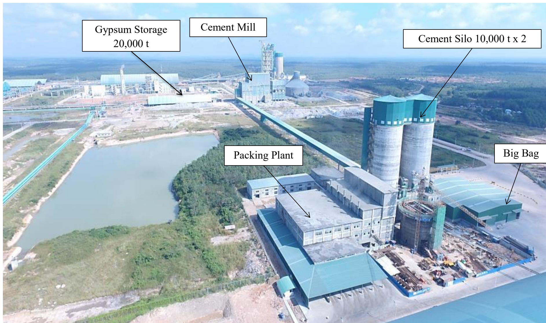
Figure 7: Plant Layout Overview of Packing Plant and Delivery Area
