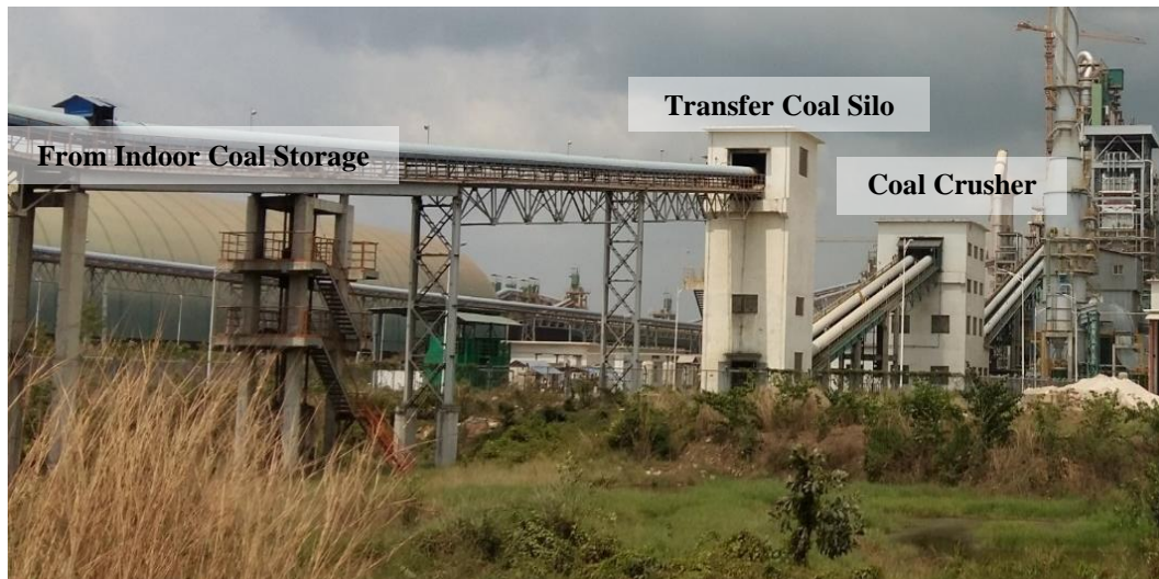
Figure 3.4-10: Coal Conveying System Used in MCL
