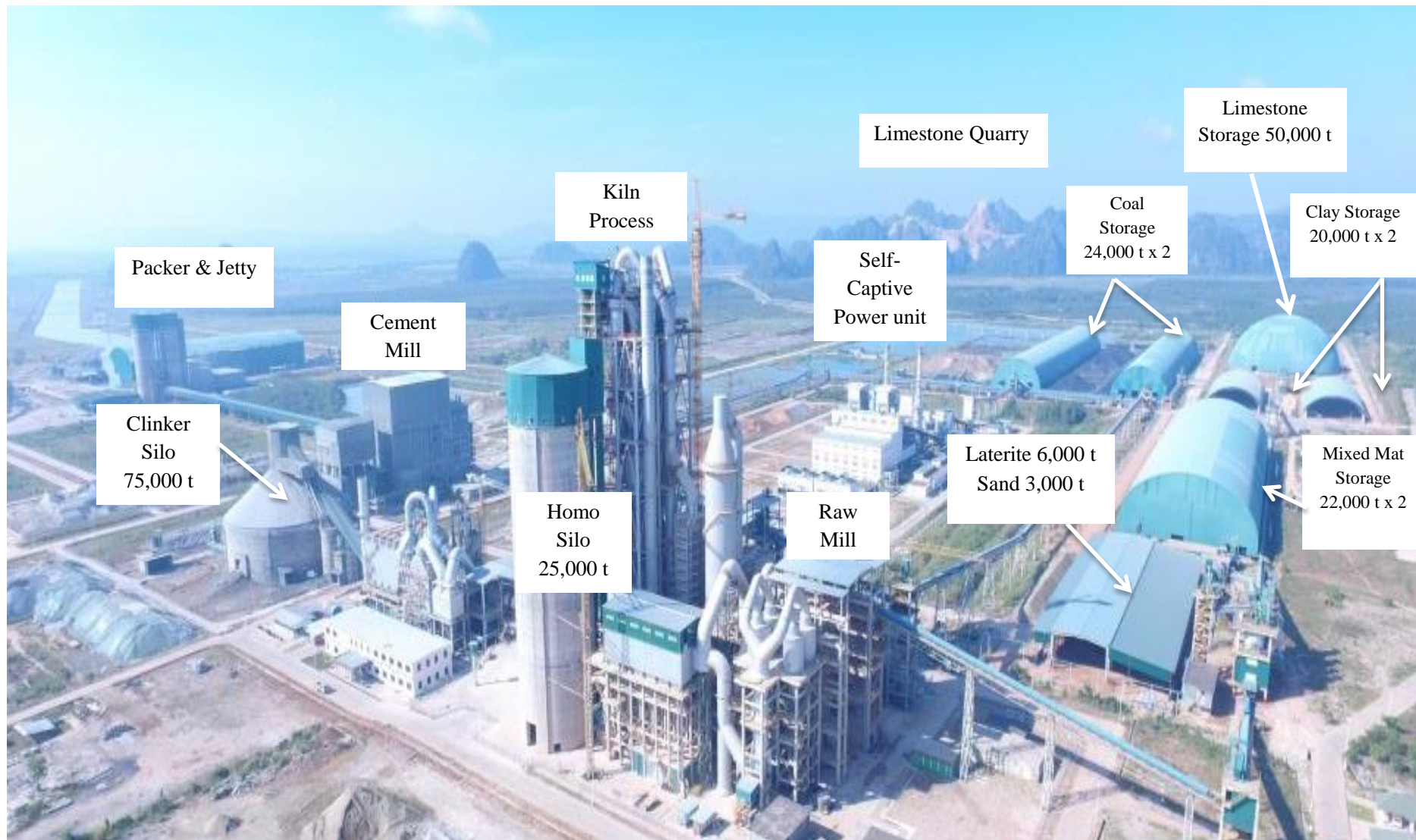
Figure 5: Plant Layout Overview of Cement Factory Compound
