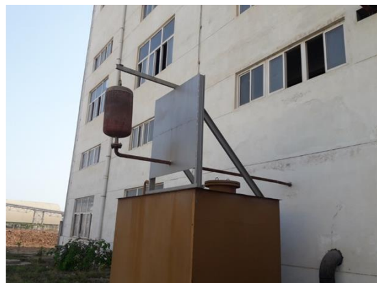
ii) Steam Blow Pipe with Silencer
