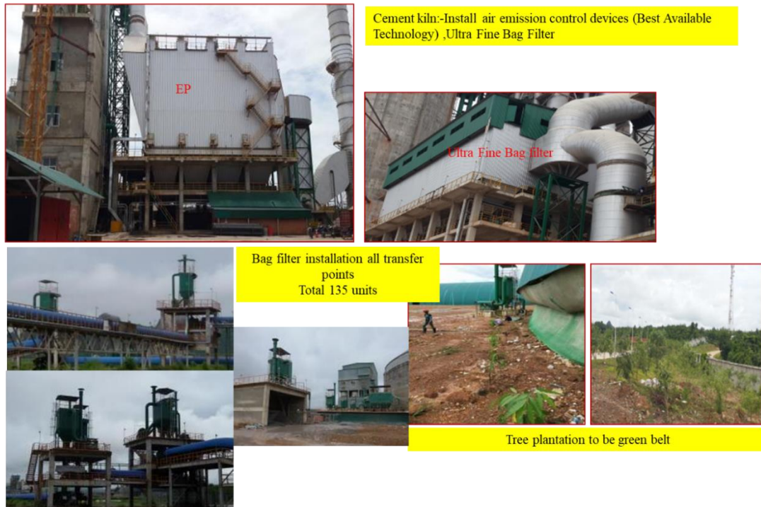
Figure 7.3-5: Installation of Dust Collectors and Bag Filters for Reduced Air Emissions
