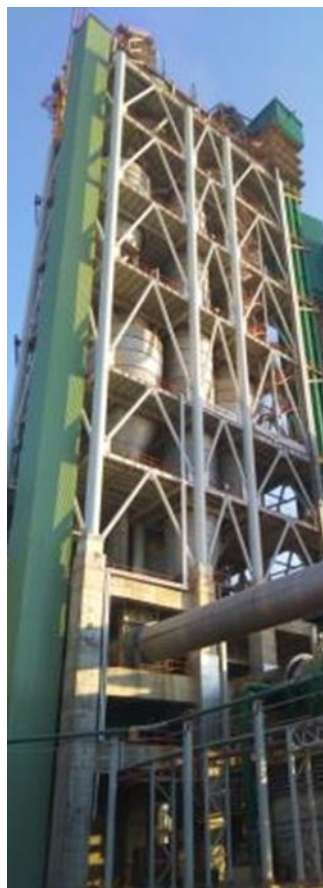
Figure 3.8-3: Kiln and Cyclone Preheater used in MCL's Cement Plant
