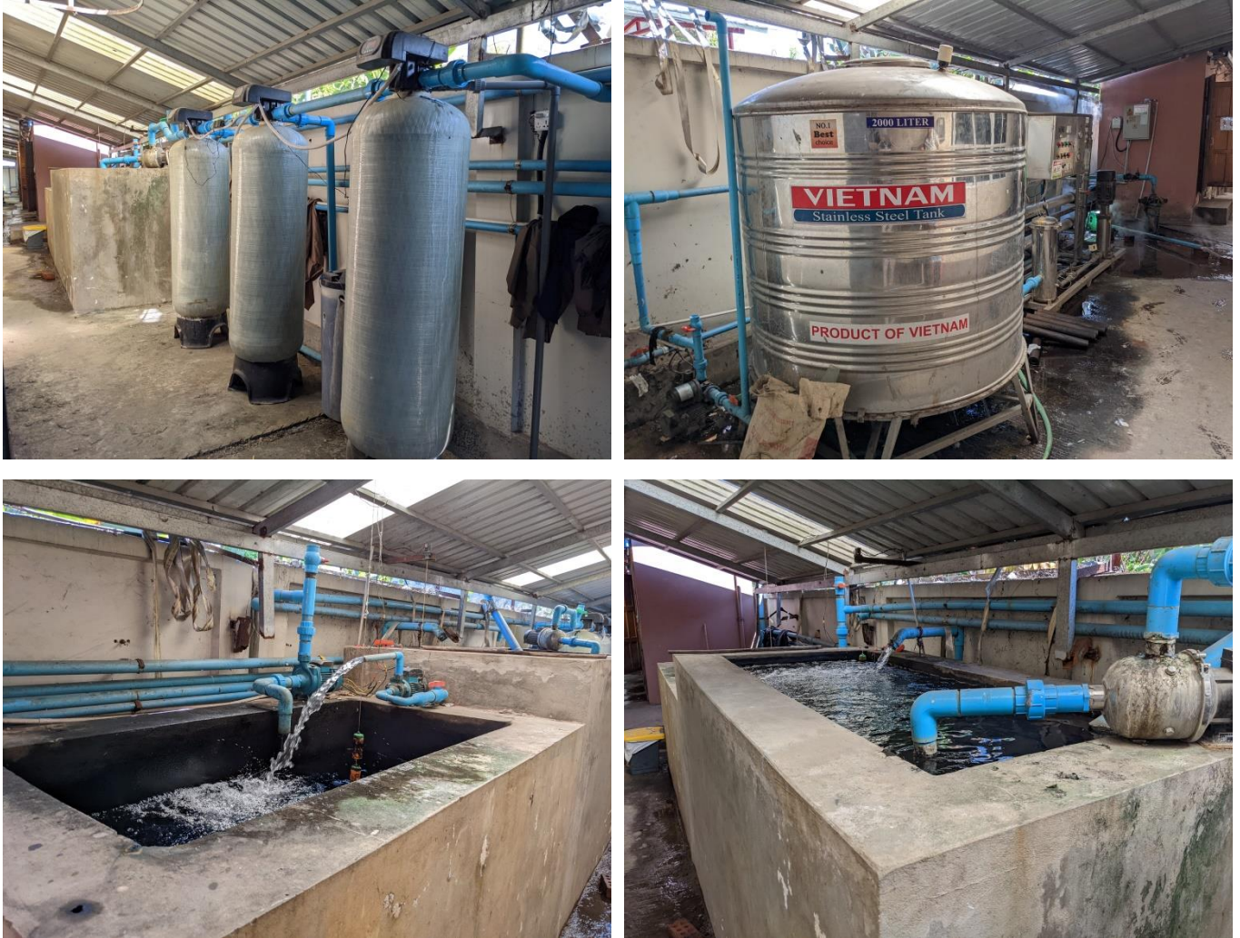
Figure 3-9 Water storage tank and drinking water supply
