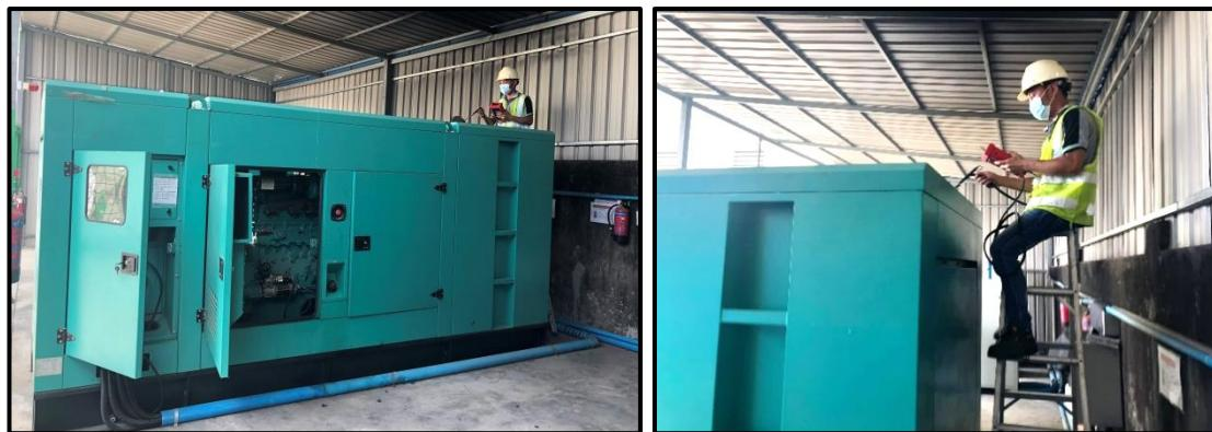
Figure 4-10 Generator Stack Gas Emission Quality Measurement
