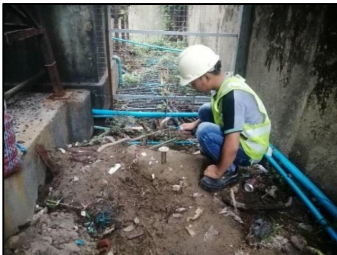
Figure 4-15 Soil Sampling for Analysis
