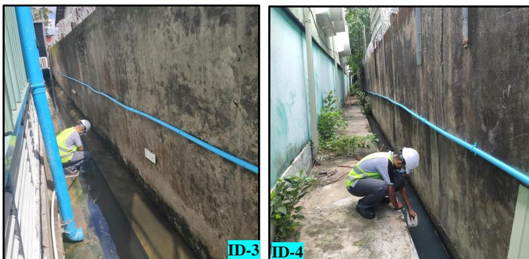
Figure 4-13 Taking Samples for Wastewater Quality Test
