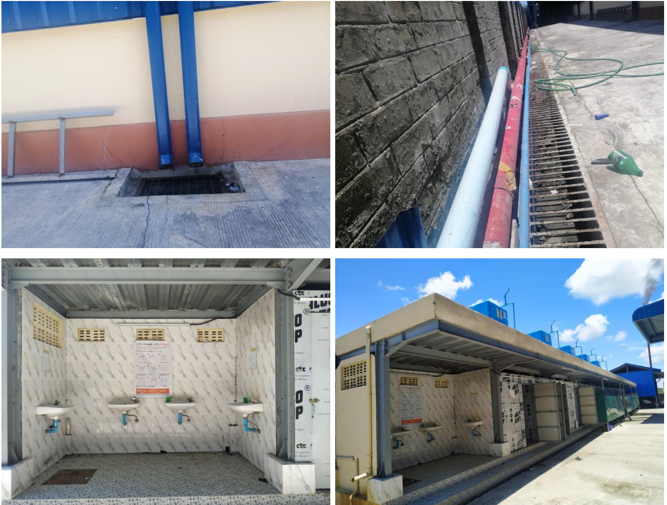
Figure 3-12 Drainage and Toilet facility
