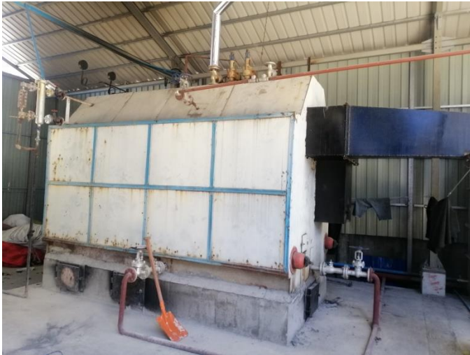
Figure 3-10 Steam Boiler
