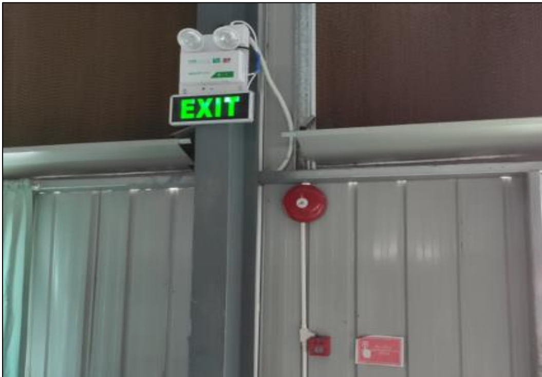
Figure 3-30 Fire Alarm
