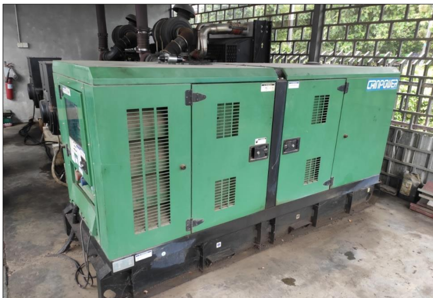
Figure 3-21 375 kVA Generator
