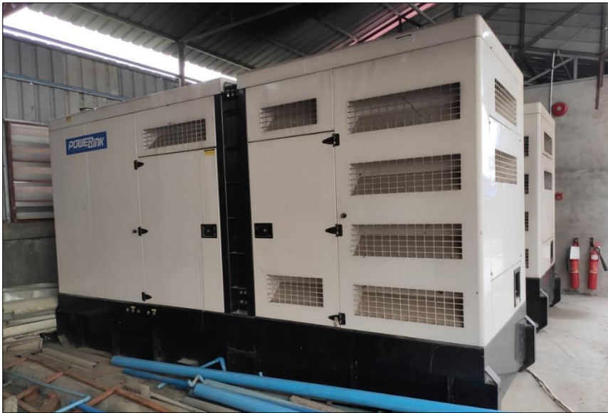
Figure 3-22 500 kVA Generator
