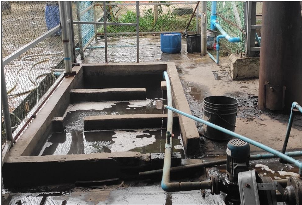
Figure 7-2 Sedimentation Tank of the Boiler Chimney
