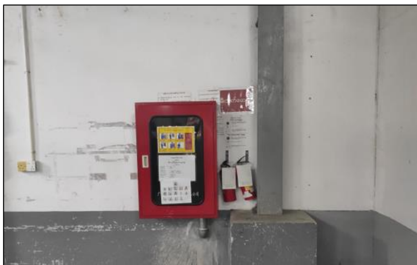
Figure 3-29 Fire Hose Reels and Fire Extinguishers
