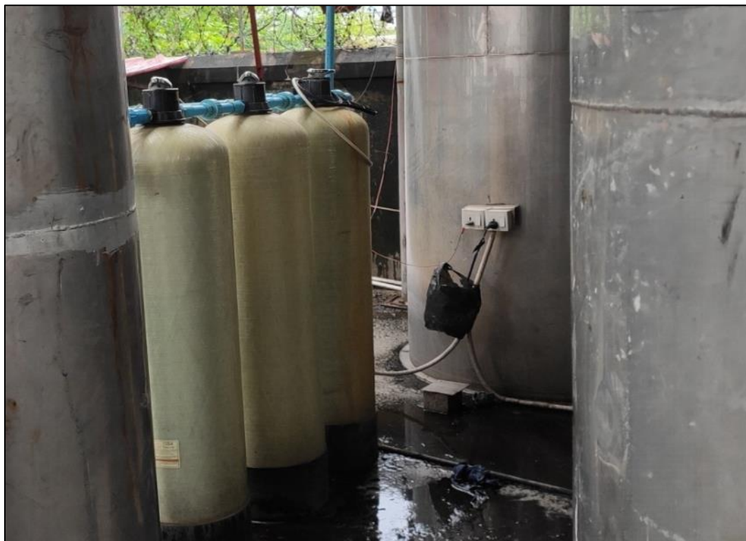
Figure 3-19 Filtering System for Water from Tube Well
