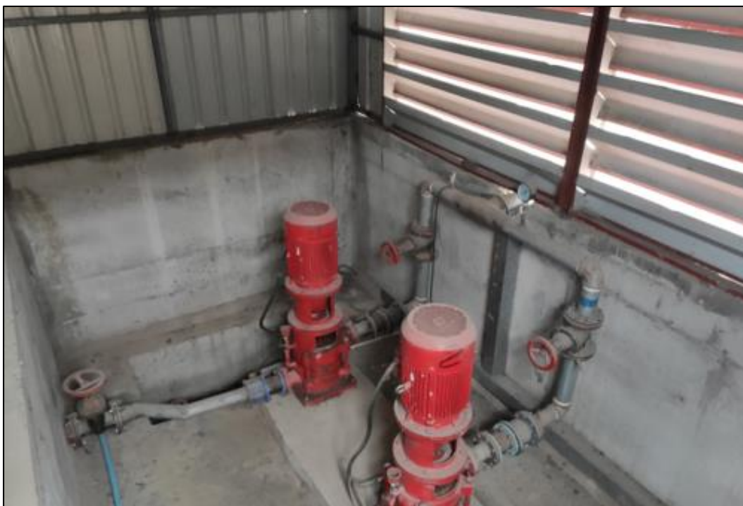
Figure 3-31 Fire Pump
