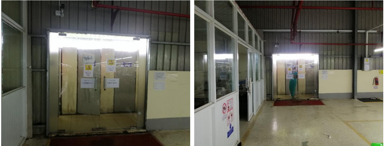
Figure 3-15 Toilet Facility Photo
