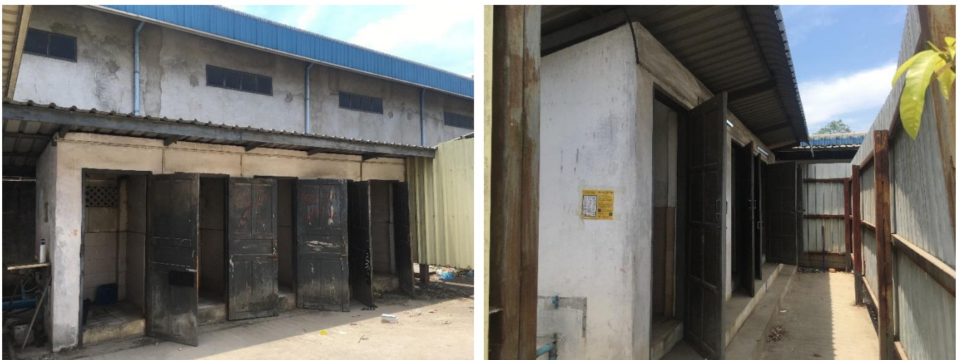
Figure 3-13 Toilet Facility Photo
