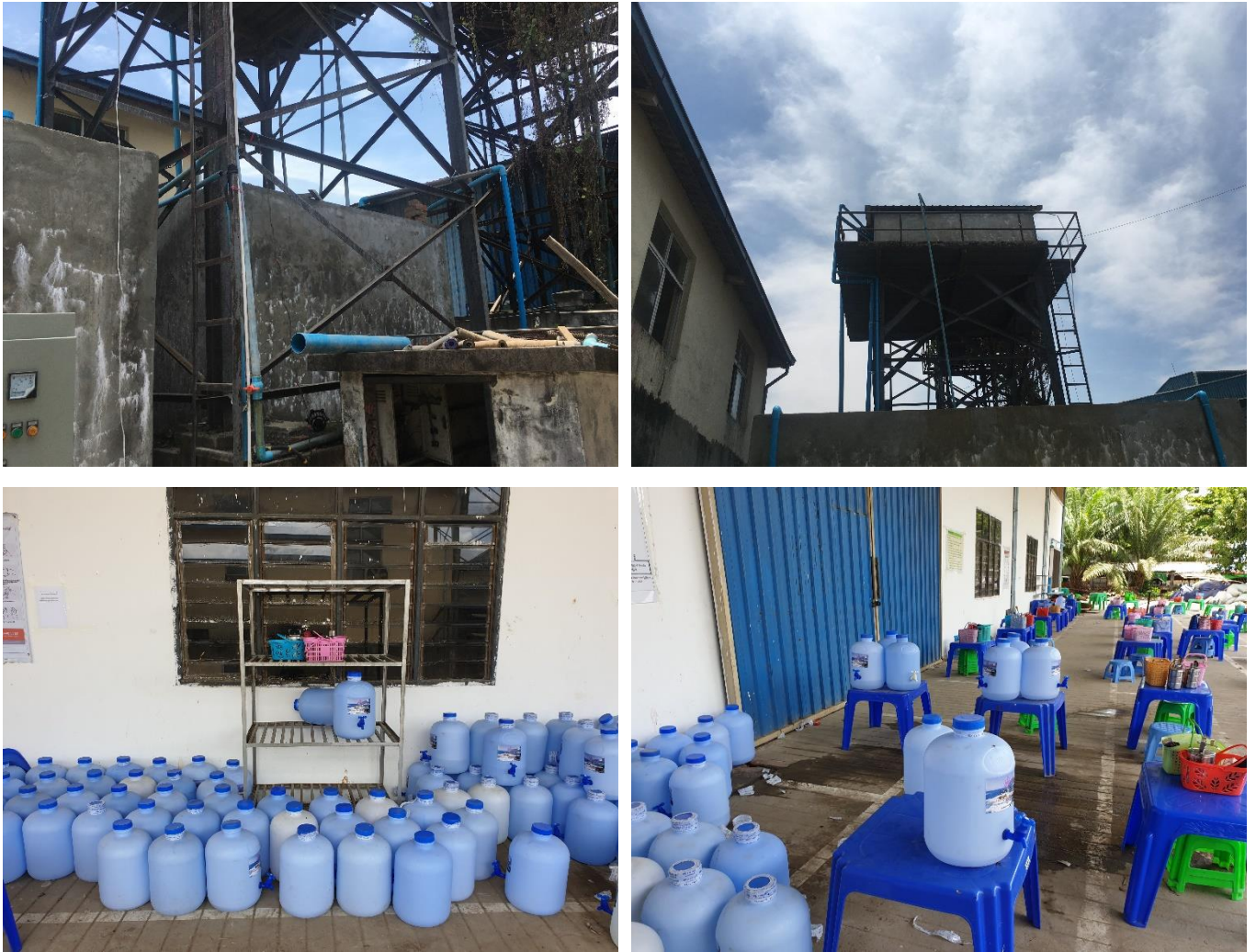
Figure 3-4 Water Storage Tank and Drinking Water Supply
