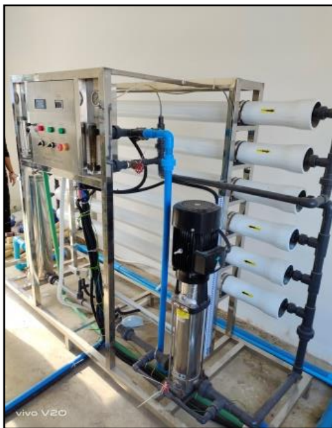
Figure 7: Water Supply (Deep Well) with R.O Water Treatment System
