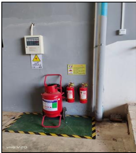
Figure 5: Fire Protection Equipment
