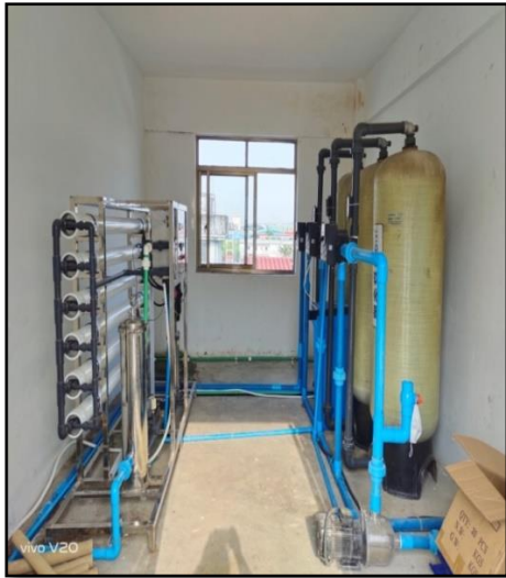
Figure 4: Water Supply with Reverse Osmosis Water Treatment System
