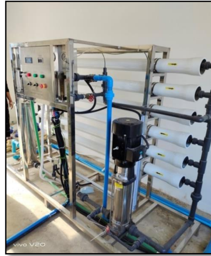
Figure 4: Water Supply with Reverse Osmosis Water Treatment System
