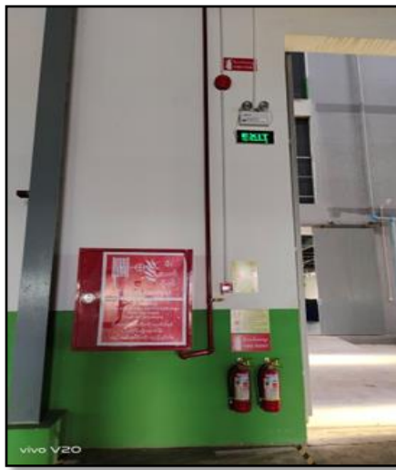
Figure 5: Fire Protection Equipment
