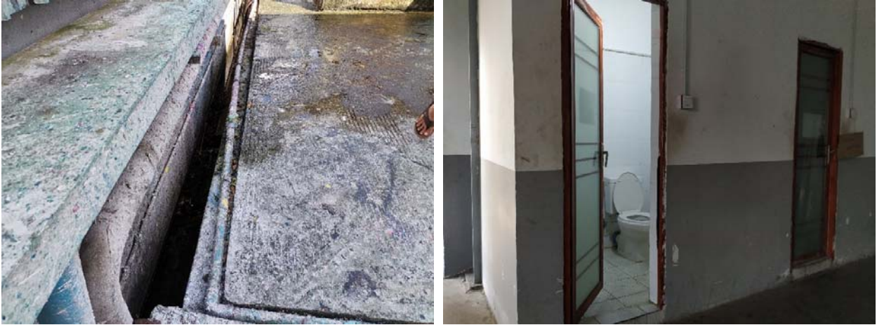
Figure 3-11 Drainage and Septic tank in project area
