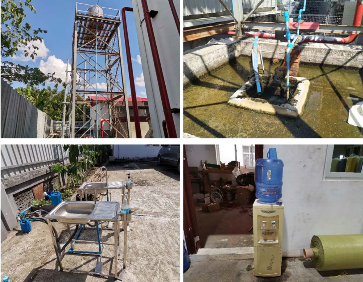
Figure 3-9 Water storage tank and drinking water supply
