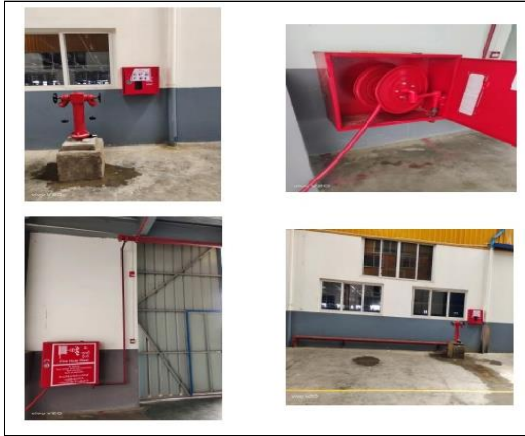
Figure 6: Fire Protection Equipment
