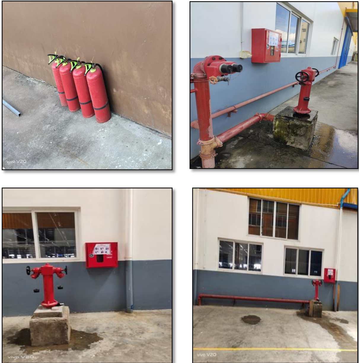
Figure 3: Fire Safety Equipments
