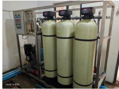
Reverse Osmosis water treatment plant
