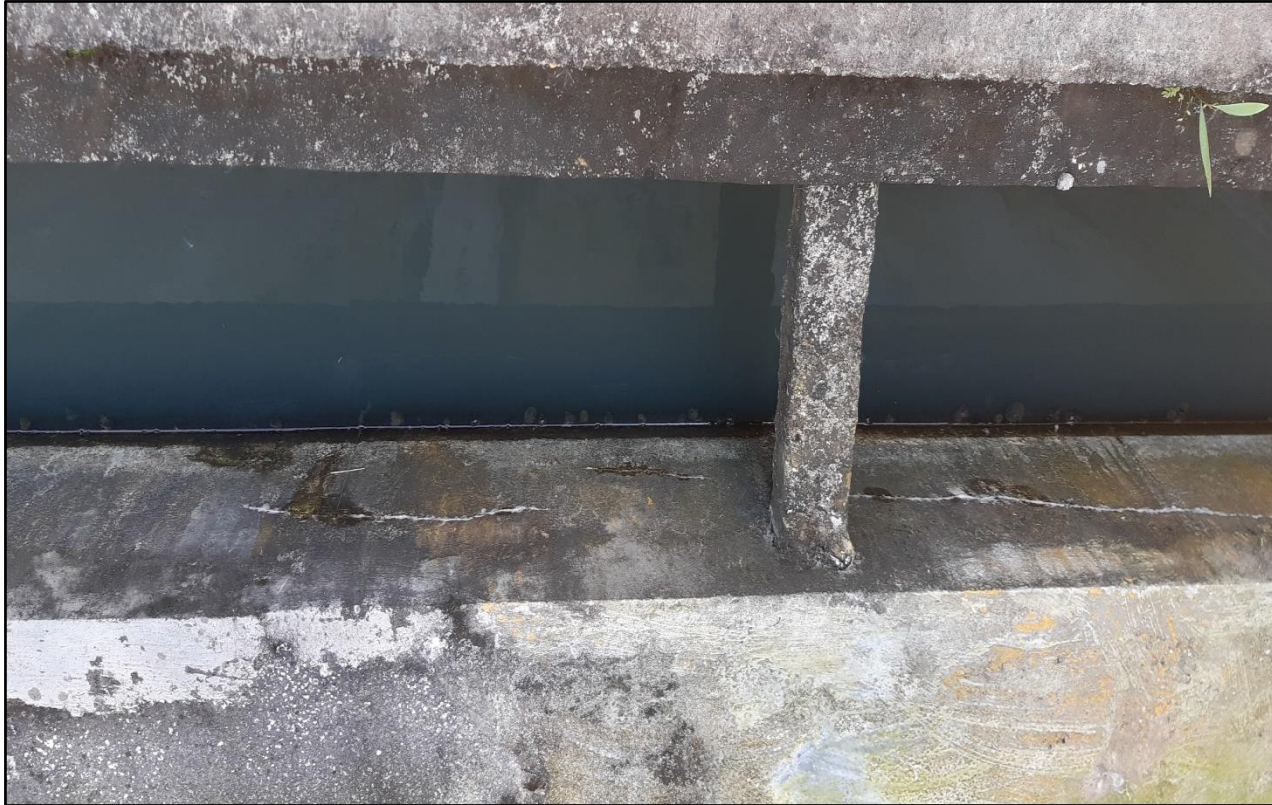
Figure 8: Masonry Drainage at Project Site
