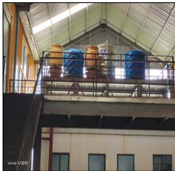
Figure 8:Water Supply (Deep Well) with R.O Water Treatment System
