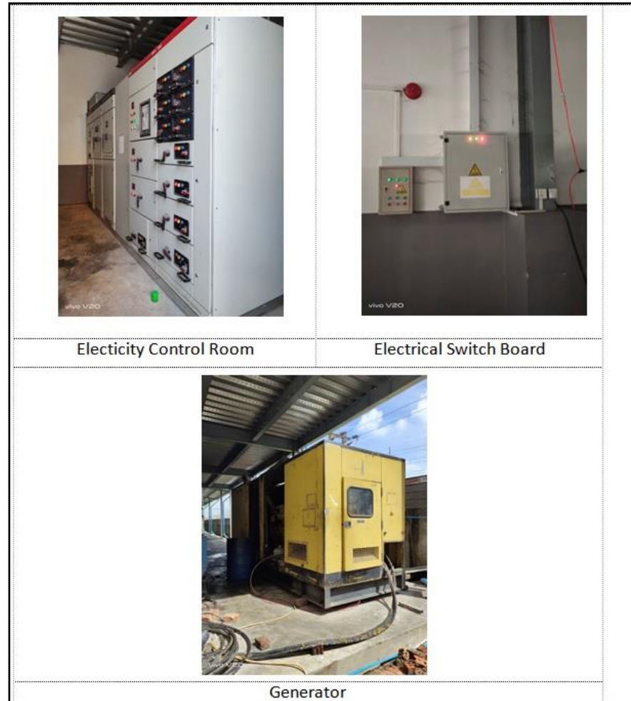
Figure 5: Electricity Control Room and Emergency Power Generation Gen-set
