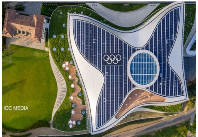
Solar Panels on Roof Top
