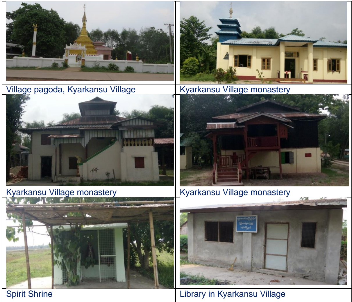
Figure 4. 70: Kyarkansu Village Buildings
