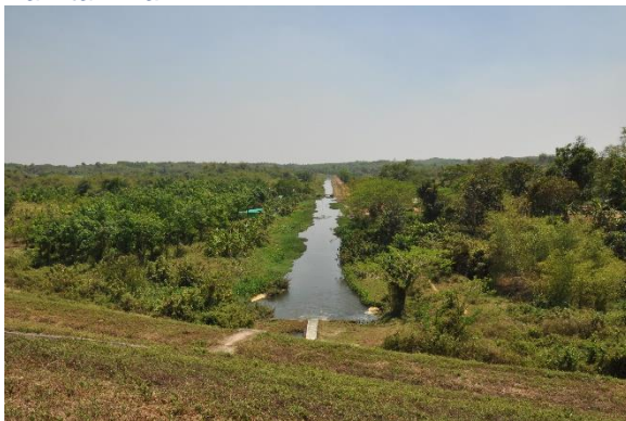
Water Channel to Agricultural Zone
