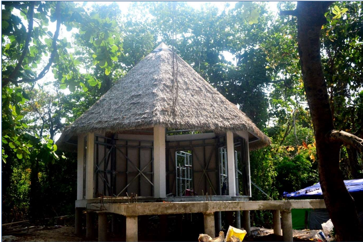
Figure 5-5 The cottages being assembled in the island
