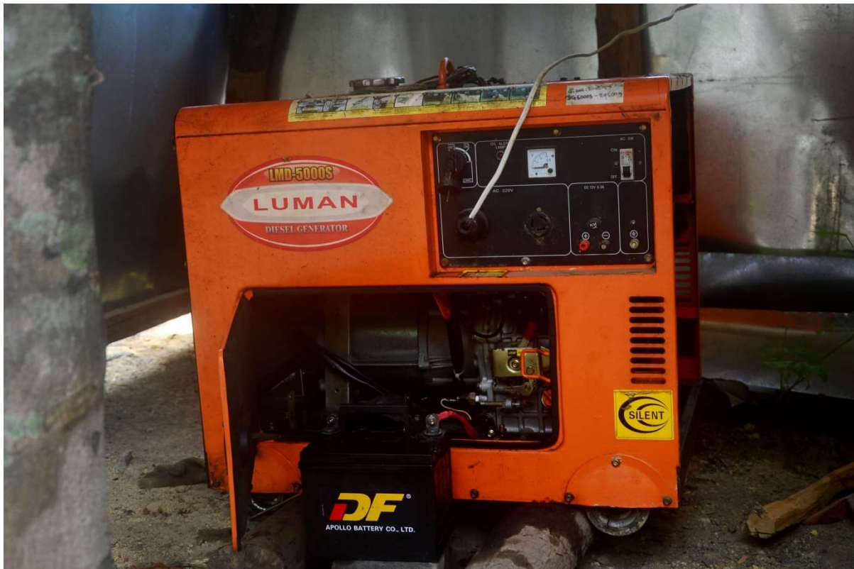
Figure 5-7 The 4.5 kW Diesel Generator used at Phoni Island
