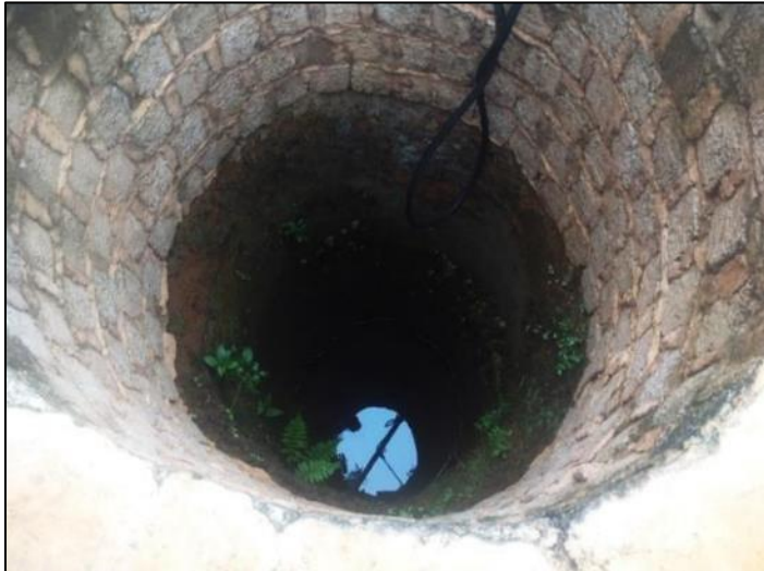
Figure 7-22: Shallow water well ending in the residual soil.
