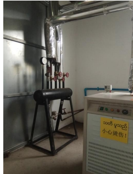
Figure 3-9 Electronic Steam Boiler at Xiang Rui Factory
