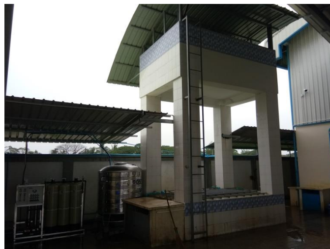
Overhead and ground water tank
